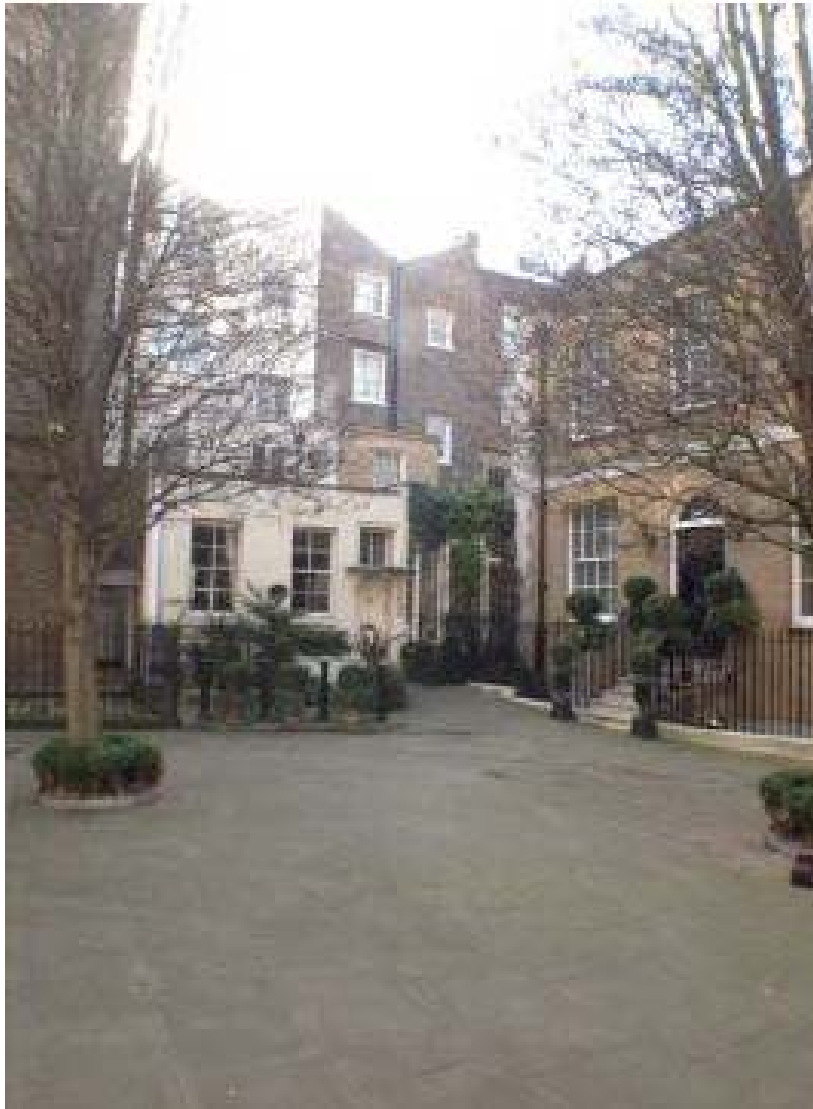
View of the rear of application property (existing brick extension) from Wyndham Place
